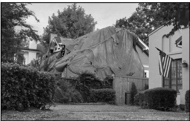
A house on Augusta Road in Greenville, owned by Kevin and Hayden Kozak, is still covered with blue tarps one year after sustaining major damage from a massive tree downed by Helene. Pictured on Tuesday Sept. 23, 2025. (Photo by Mark Susko/Special to the SC Daily Gazette)
